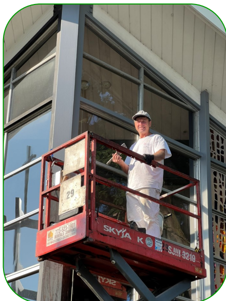
JSB Painting LLC begins cleaning and painting the rusty metal beams at the entrances to the church.
