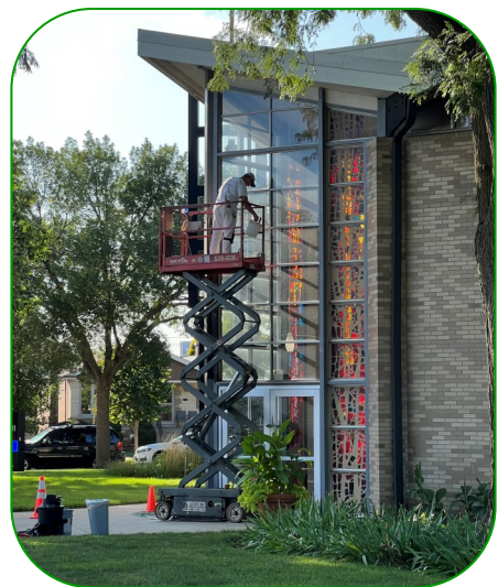
JSB Painting LLC begins cleaning and painting the rusty metal beams at the entrances to the church.
